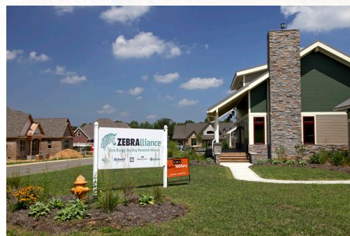
ORNL research houses serve as realistic residential test beds
